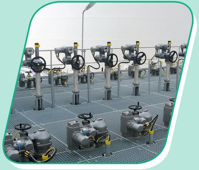
*In a modern storage facility of petroleum products, on average several hundred – maybe thousands – of valves are installed. Electronic actuators are used for their handling, allowing them to perform the necessary manoeuvres without the physical presence of personnel.*
